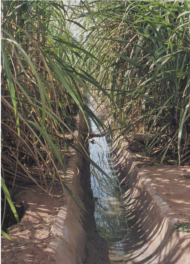
Figure 2–2. An irrigation canal in the Zimbabwean lowveld, where transmission is intense. To keep the canal from becoming a breeding site, it must frequently be flushed and permitted to dry out. (Courtesy of D. Stürchler.)
